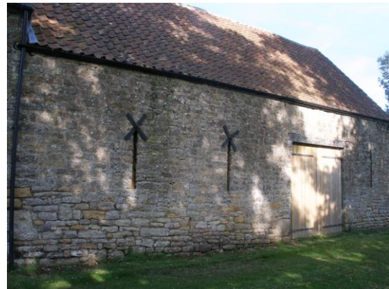
Fig.51 Barn at Innage Farm. Its recent conversion retains its slit openings with internal timber shutters
