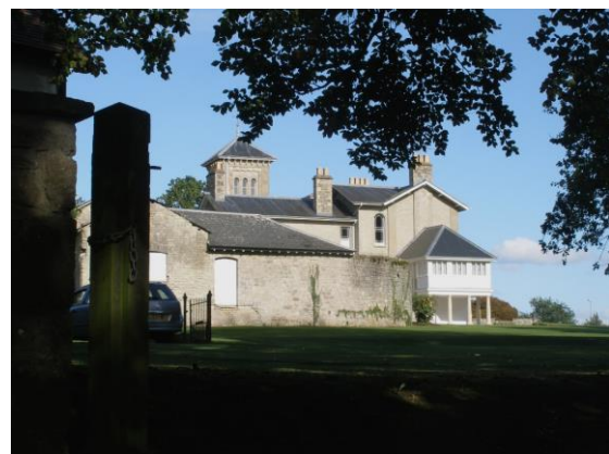
Fig.57 The Italianate tower, low pitched roofs and projecting eaves of St Tewdric's, preside over its extensive countryside setting. The later timber viewing gallery on the corner of the building enhances its simplicity
