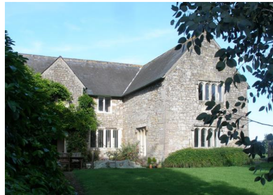
Fig.50 Innage Farmhouse. A fine medieval building demonstrating its prosperity by the use of numerous stone mullioned windows and entrance bay
