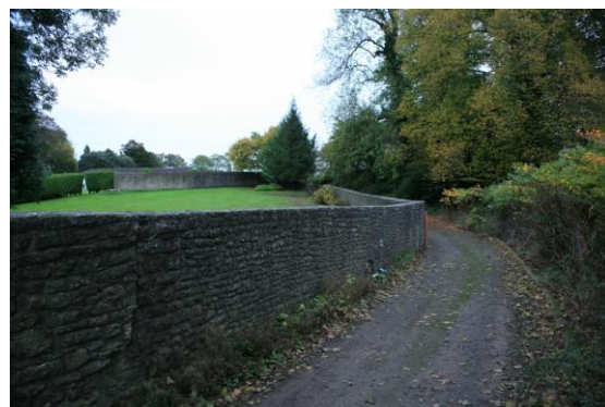
Fig.69 Curving stone walls create dynamic lines in the landscape and create positive and comfortable enclosure particularly to roadsides
