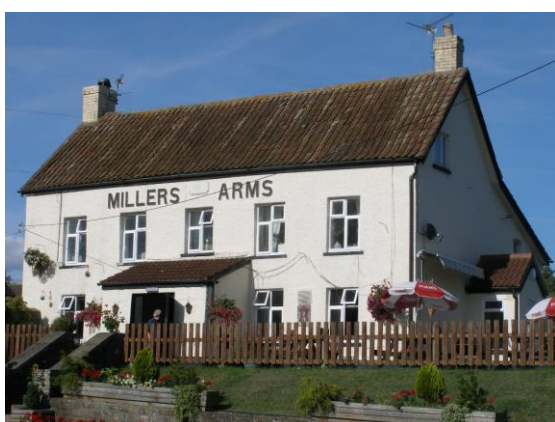
Fig.54 The Millers Arms Inn retains its vernacular character with gable end chimneys and single-storey 'catslide' roof extension to the rear. The large porch is probably a later addition
