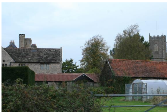
Fig.67 Clay pantiles to Mathern Palace outbuildings
