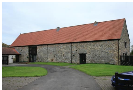
Fig.13 The large converted tithe barn and outbuildings have a strong presence on the roadside
