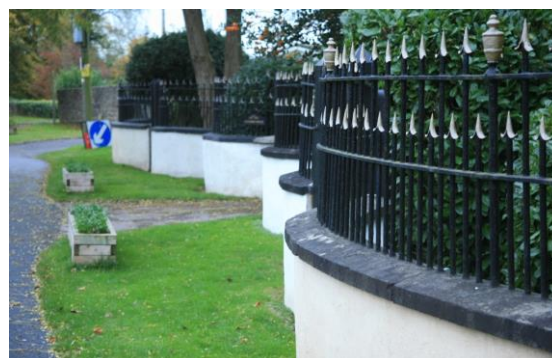
Fig.22 Curving walls to Mathern House are a striking feature in the conservation area
