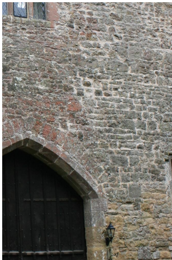
Fig.64 Typical stone treatment to walls in the conservation area
