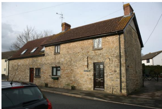
Fig.27 A former barn, Shop Cottages, displays typical treatment of random rubblestone walls
