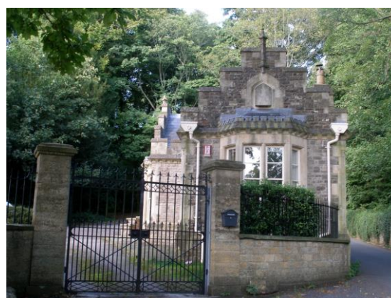
Fig.60 The neo-Jacobean design of the Lodge to 'Wyelands' is a lively composition of battlemented parapets, crowstep gables and a mullioned oriel
