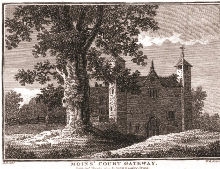
Fig.4 Moynes Court gateway by R.C. Hoare c1800
