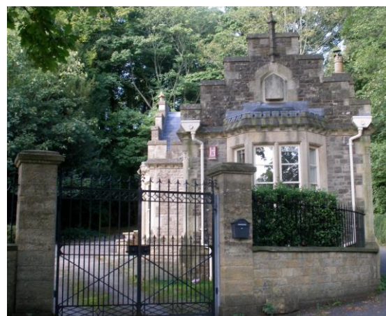
Fig.33 Lower Lodge – this Jacobean style lodge marks the south entrance to Wyelands estate
