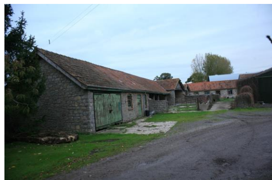
Fig.16 Double Roman interlocking clay tiles are a feature of farm buildings including those at Innage Farm
