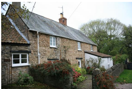
Fig.66 Natural slate remains on many buildings including Moynes Cottage
