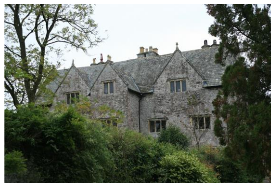
Fig.12 The 17 th century Moynes Court with attractive gables and large relieving arches above stone mullion windows
