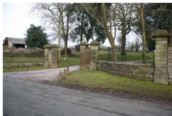
Fig.40 St Tewdric's use of Forest of Dean stone extends to its boundary walls and gate piers
