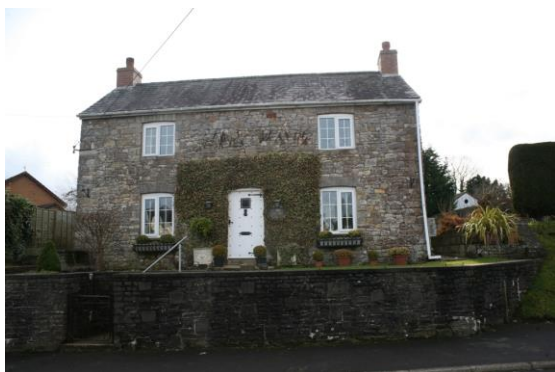
Fig.24 Old School House, raised above the roadside, maintains the building line with other properties located close to the road
