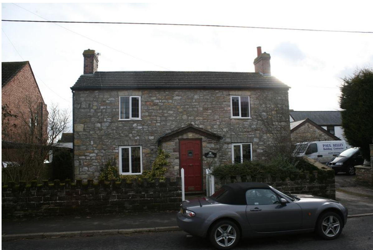
Fig.74 Rose Cottage; Modern roof coverings and modern porch and door have eroded the traditional character of this cottage but these changes are reversible
