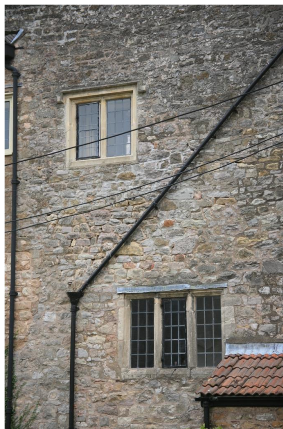
Fig.14 Rubblestone and Bath stone dressings to Moynes Court
