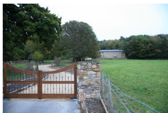
Fig.42 East Wood forms a background to the house
