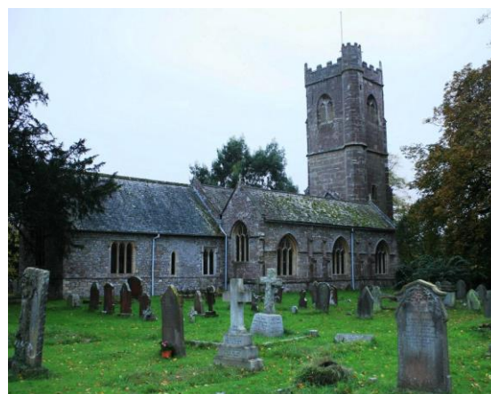
Fig.49 St Tewdric's church. A mainly 14 th century building including a graceful tower. Its relatively large size is due to its relationship to the adjacent Bishops Palace. The church was extensively restored in the 19 th century
