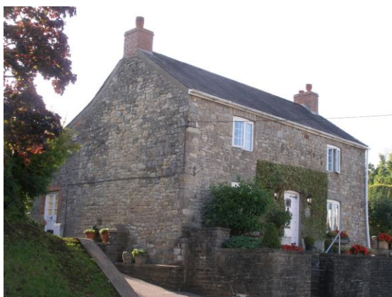
Fig.53 The 'Old School House' is a well preserved vernacular building. Its stonework, including voussoirs over the windows, are well constructed
