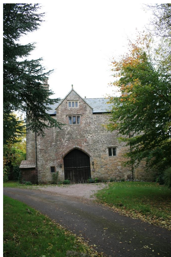
Fig.73 The bulk and scale of the stone gatehouse terminates views along the driveway to Moynes Court
