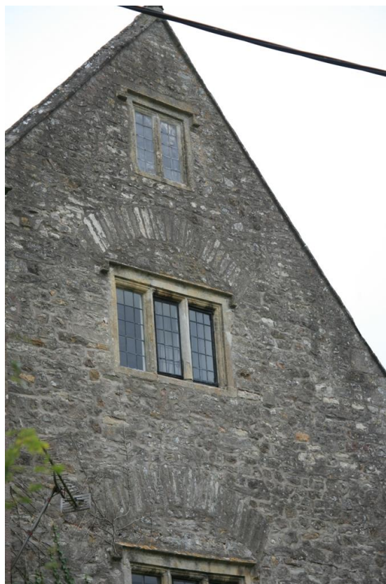
Fig.65 Stone mullion windows to Moynes Court reflecting the higher status of this house
