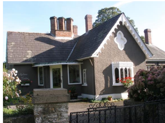
Fig.56 The 'Gothick' inspired cottage ornée style of the early 19 th century is apparent in the multiple angled chimneys, decorative bargeboards, quatrefoil gable decoration and the mullioned oriel window of Mathern Lodge
